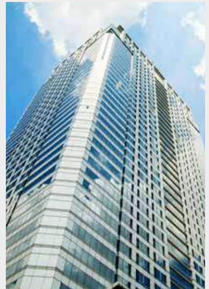
• BUILDINGS Kitting Telecom Solutions for Roof Installations
