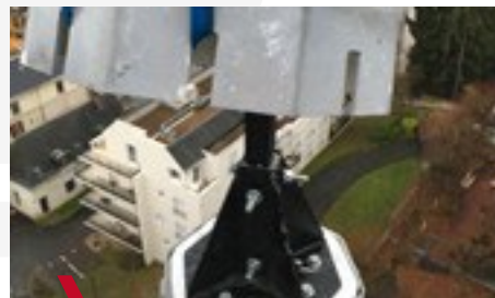
2 Installation of the new composite cross on the existing sleeve.
