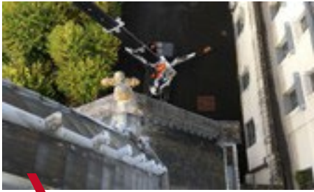
1 Access to the top by aerial platform
