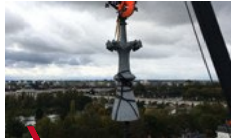
2 Dismantling of the various elements
