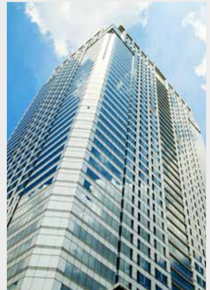
◦ BUILDINGS Kitting Telecom Solutions for Roof Installations
