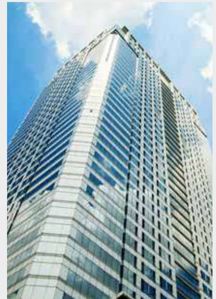
◦ BUILDINGS Kitting Telecom Solutions for Roof Installations
