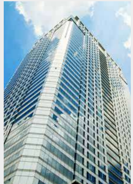
◦ BUILDINGS Kitting Telecom Solutions for Roof Installations
